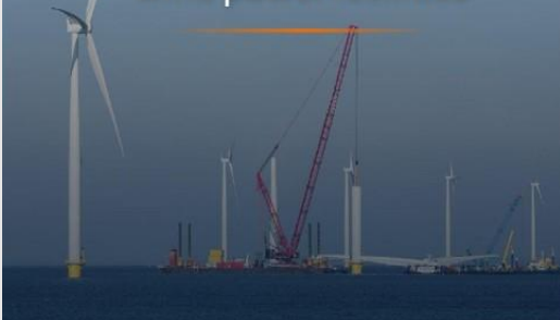
Inspection of offshore wind power facilities
